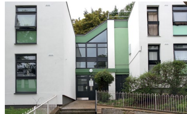
L&Q, Lewisham System: webertherm XM with webersil TF finish Client: L&Q Specifier: Faithorn Farrell Timms Contractor: Mulalley & RR Richardson Limited Applicator: ECL Contracts
