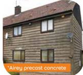
building methods, most of which were constructed between 1939 and the 1970's and were built for speed and economy of construction and not for thermal efficiency.
