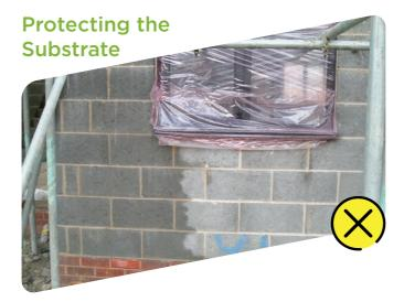
Once the blockwork has been built and is awaiting rendering, temporary guttering socks should be used to direct rainfall from areas of the wall.
