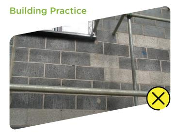
Infilling or coursing with dissimilar materials should be avoided. Different types of blocks expand and contract at different rates creating increased stresses which can
