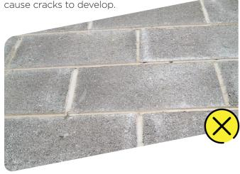
Blockwork should be laid in a regular brick bond pattern and perp joints should not clash. Ideally mortar joints should be finished flush, removing the risk of different thicknesses of the render which may cause 'grinning' of the blockwork through the monocouche.
