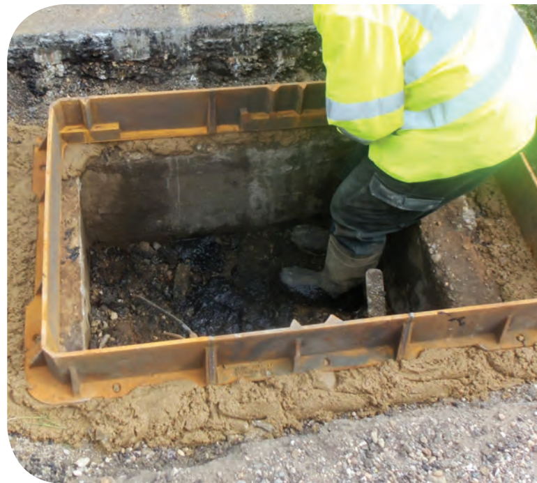
webertec bedding mortar haunching
