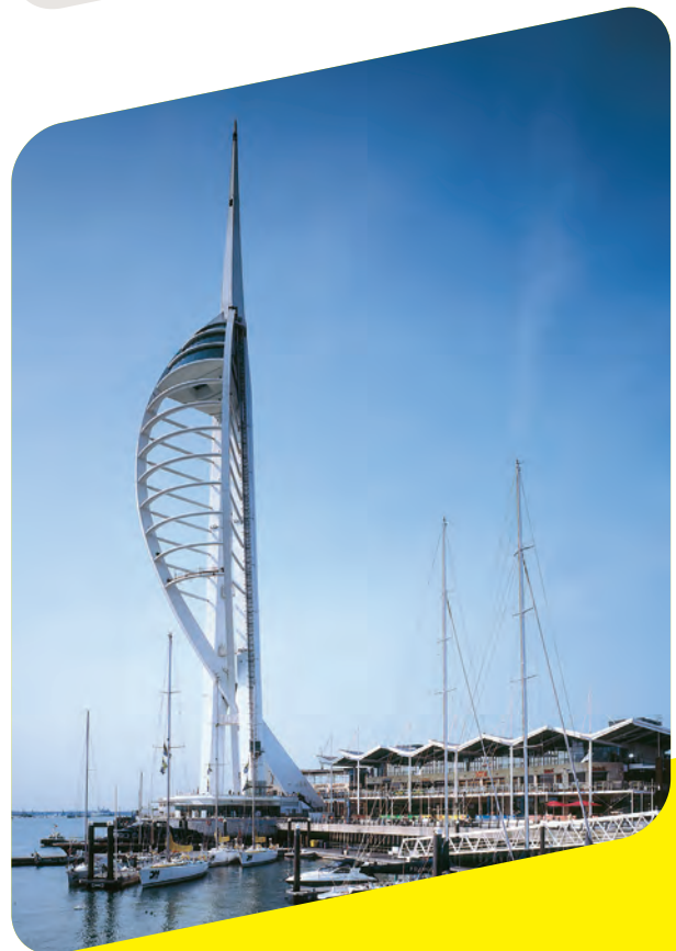
Spinnaker Tower, Portsmouth. webercem grout and webercem precision grout
